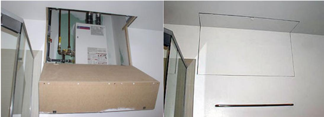
The pictures above show a gas unit that is supplying two full bathrooms, a kitchen and laundry room. The unit is hidden behind an access door in a recess in the master bathroom.
